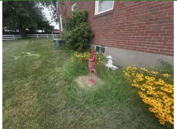
Photo 8 - View of the hand well on the eastern end of the residence on the site
