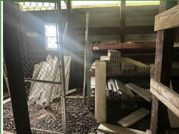
Photo 7 - View of the interior of the larger shed on the site
