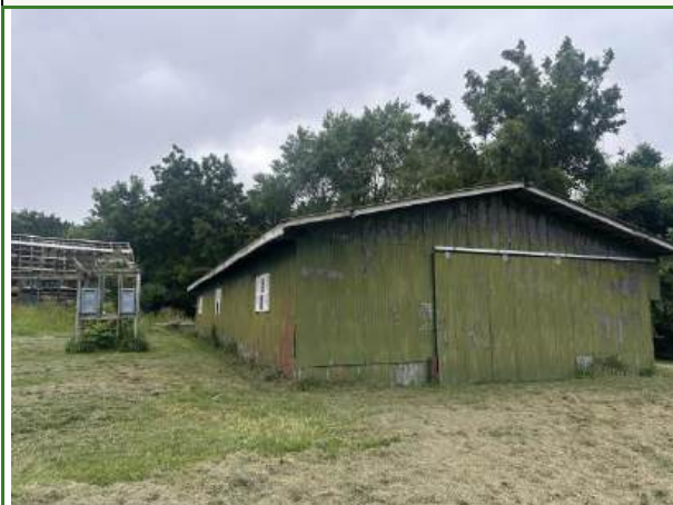
Photo 5 - View of the larger shed on the site
