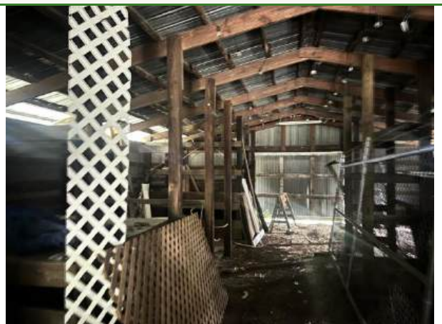
Photo 6 - View of the interior of the larger shed on the site
