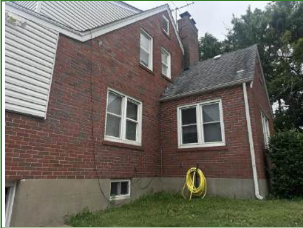
Photo 1 - Overview of the west end of the residence on the site
